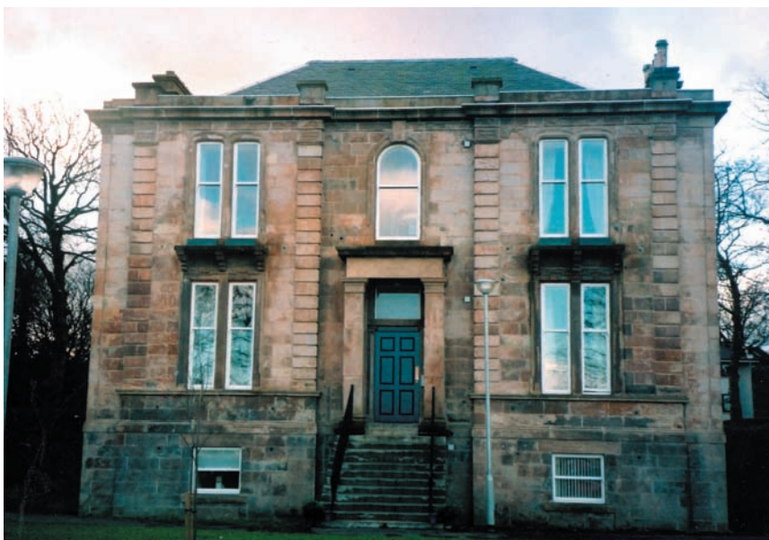
Netherkirkton House, after refurbishment ▼
