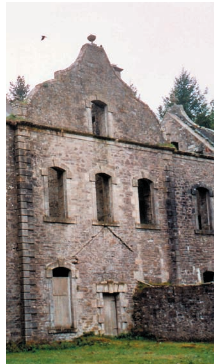
Detail, Carmichael House, Thankerton ▲
