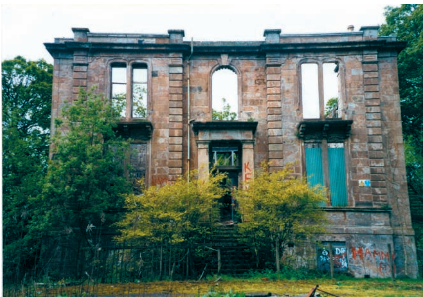
Netherkirkton House, before refurbishment ▼
